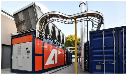
Startup AtmosZero installed its first steam heat pump, the brightly colored container shown above, as part of a pilot project at the New Belgium brewery in Fort Collins, Colorado, in June.
